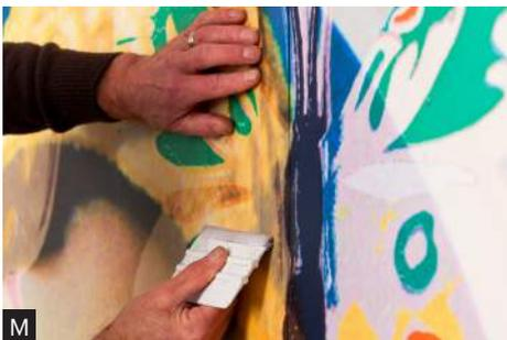
Fix the first drop from the right hand side, making sure the left hand edge of this drop aligns with the vertical line. This is the most critical point and this first panel must be vertical to the plumb line. Smooth out any bubbles or ripples with a brush or your squeegee, in a vertical direction only. Wipe off any excess paste with a damp sponge.
